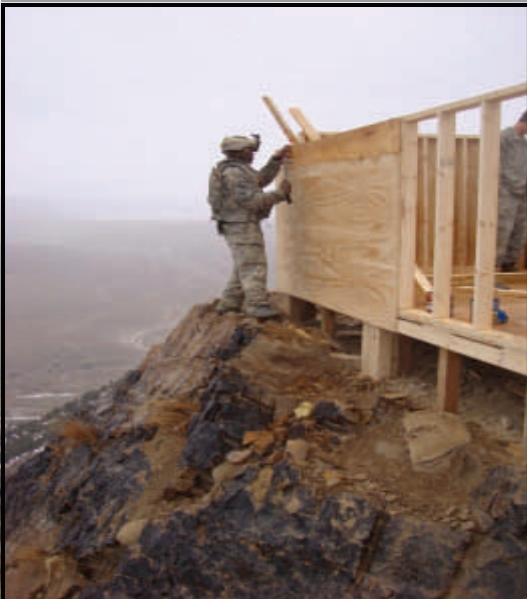
Mountaintop Duty Photo by Capt. Nicholas Melin January 25, 2008 Sgt. Carlos Bell nails the wall for a bunker.
